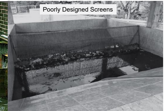
Inclined screens | Perforated tough | Access for operator to rake the screens
