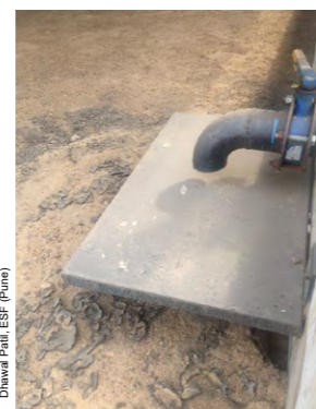
Use of splash plate to reduce erosion and even spreading of sludge
