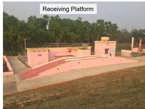
Clear access to the receiving station Easy manoeuvring of trucks pre and post decanting
