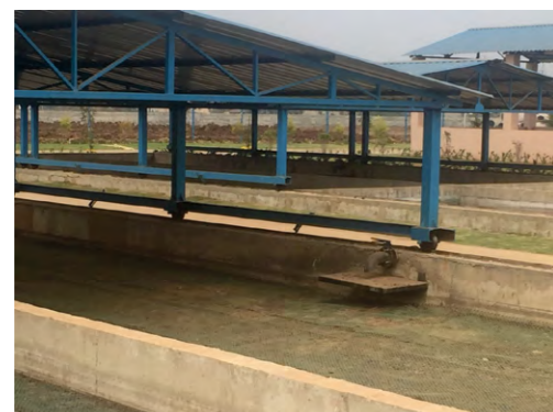
Easy access to valves from outside of the bed
